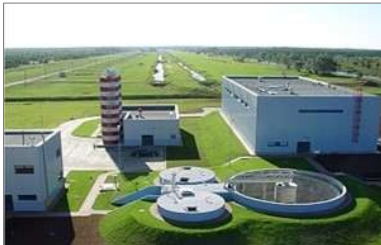
4.12.2.3.1 Fig. Klaipėda City Water Supply Area No. 3
